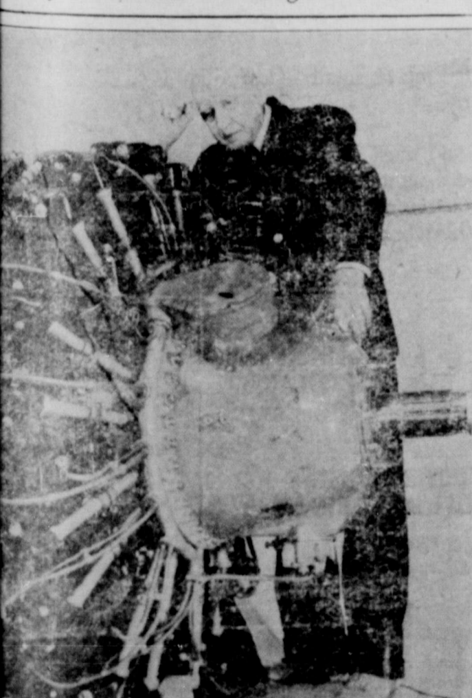
MEMPHIS, Mich.—Memories of mechanical heartbreaks at Kitty Hawk returned for 73-year-old Charles Taylor (above) as he this 2,000-horsepower airplane the Ford Rouge soon will produce for the sand dunes of Kitty Hawk, N. C. He said the Wright plane was driven by a 200-pound engine that turned up only 12 horsepower. This mechanical giant weighs 2,350 pounds. Ford is rushing toward completion a $27,000,000 plant in which these powerful Pratt & Whitney engines will be built.
