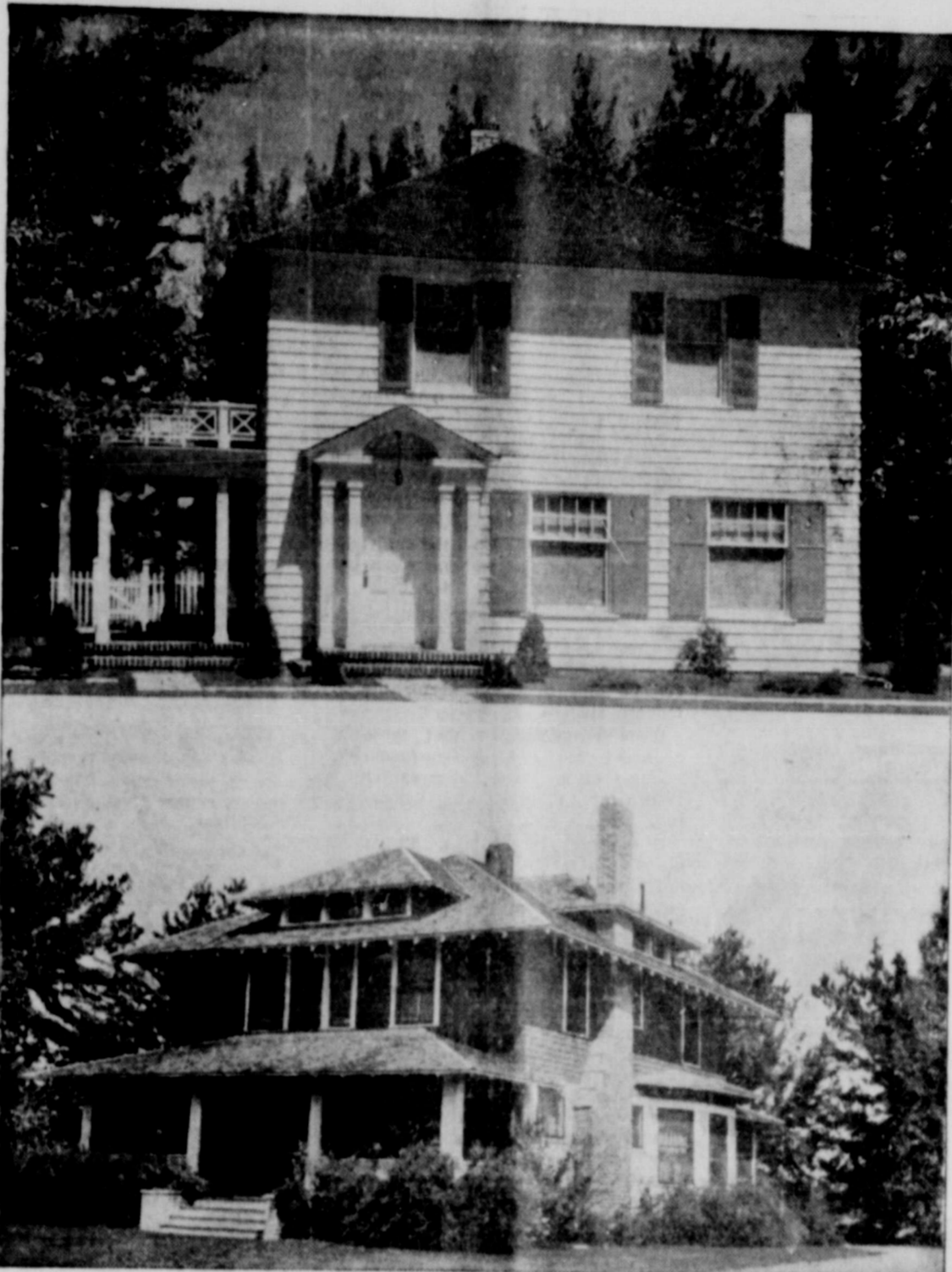
The transition here from a dated dull-appearing house to a bright Colonial-type home of permanent appeal seems almost an act of magic. Actually it is a relatively simple modernization treatment, representing the kind of value-restoring work going on in the older sections of virtually every city in America.
