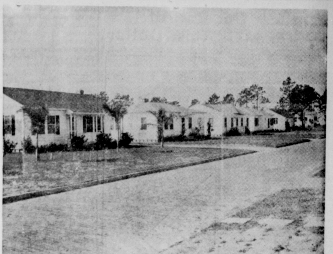
The attractiveness of this new neighborhood is likely to be lasting, largely because of the desirable features which have been built into it, according to Federal Housing Administration Land Planning officials. Neatly paved and curbed streets, generous set-back of buildings, preservation of existing trees, and planting of the grounds provide a fitting complement for well-designed houses. Maintenance is less costly and results more satisfying where street improvements are installed in a permanent manner and their cost included in the sale price of the completed property.
