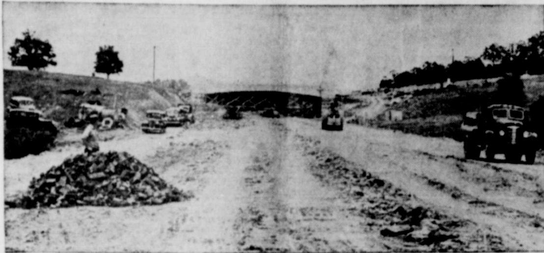
As many as 15,000 workers have been employed at one time on the four-lane superhighway between Harrisburg and Pittsburgh, which is producing an estimated 20,000,000 man-hours of work. The construction of the highway is being financed by a loan of $40,800,000 from the Reconstruction Finance Corporation and a grant of $29,250,000 from the Public Works Administration. Providing low grades and easy curves through the Appalachian Mountains, the turnpike will extend about 162 miles. A typical highway bridge crossing over the Pennsylvania Highway is shown above.
