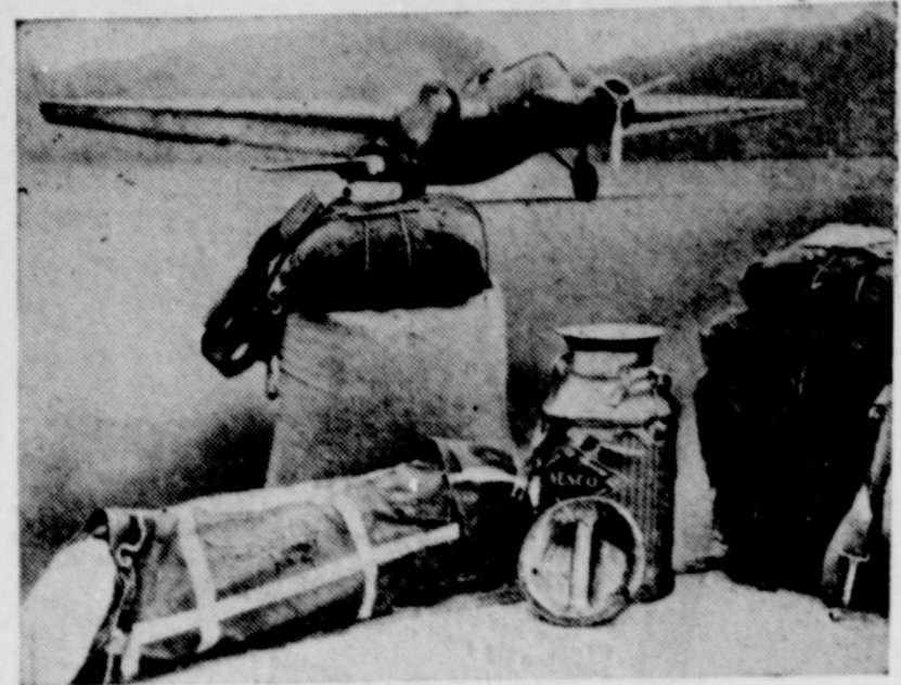
Emergency rationing of troops by airplane and parachute was successfully accomplished in Texas by the army air corps during maneuvers. This picture shows metal food container for personnel rations, bale of hay and a 136-pound sack of oats, with parachutes attached, ready to be loaded on the bomb racks of the Martin bomber, seen in background.
