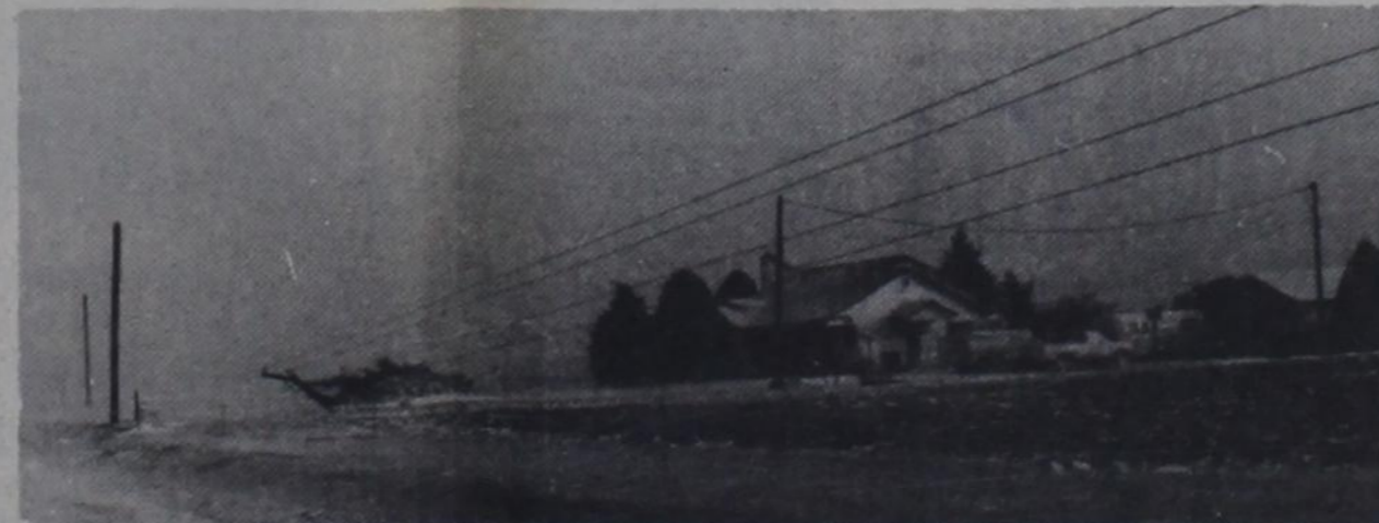
Al Gibbs home isolated by blown-down power lines Friday morning
