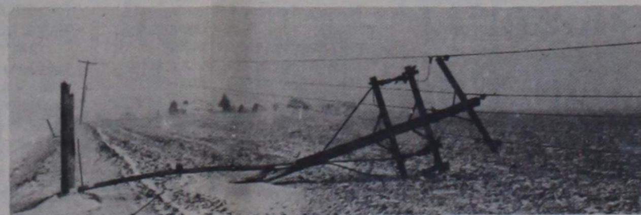
Highline pole snapped off south of Dimmitt
