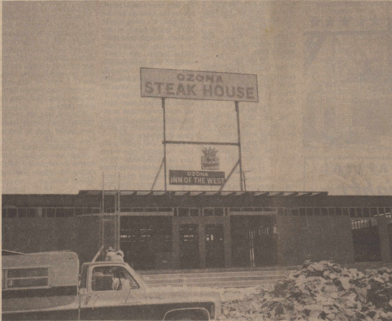
OZONA INN OF THE WEST presently under construction at 14th Street and I-10 access coming into Ozona from the east is due to open November 15. The motel complex will have 68 units in all. Eighteen units will be built above the steak house shown here and 50 units in the Inn to the east. The complex will feature a steak house restaurant, dining
