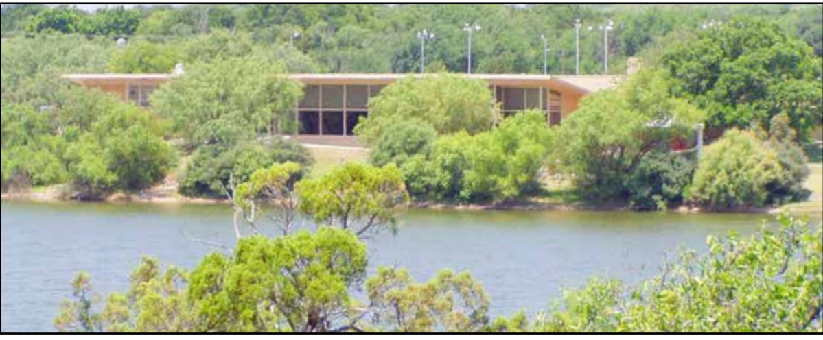
HERALD file photo The photo above shows a view of the Dora Roberts Community Center with the Comanche Trail Lake right below.
