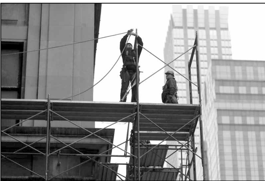
In this Feb. 20, 2018, file photo, construction workers work in midtown Manhattan in New York. U.S. productivity grew at an annual rate of 0.7 percent in the first three months of 2018, a weak reading but a slight improvement from the previous quarter.
