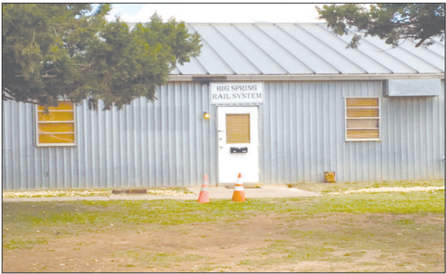
The photograph above shows the Big Spring Rail System building.
