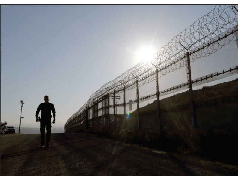
AP photo In this June 22, 2016 file photo, a Border Patrol agent walks along a border structure in San Diego, Calif. The Trump administration has proposed spending $18 billion over 10 years to significantly extend the border wall with Mexico. The plan provides one of the most detailed blueprints of how the president hopes to carry out a signature campaign pledge.
