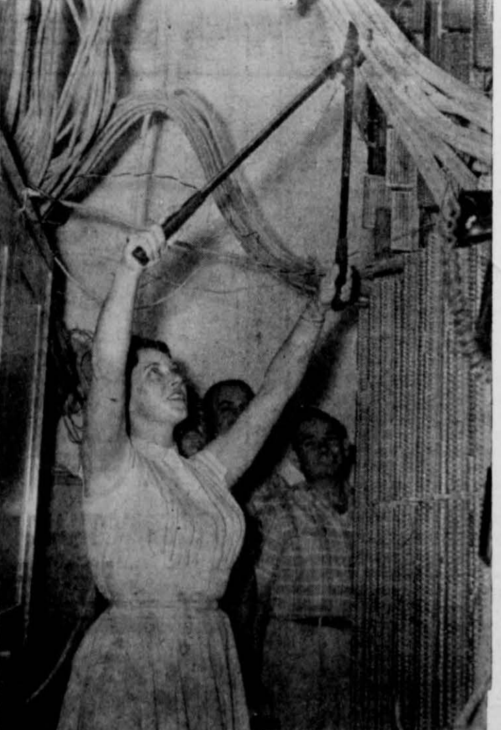
NO GOOD NO MORE —Mrs. Glenn Stiff, who was formerly Juanita Singer, was given the honor of taking pruning shears to the old telephone switchboard cables to signify the switchover to dial shortly after midnight Tuesday morning. Mrs. Stiff is the daughter of T. A. Singer, operator of West Texas Telephone Company until his death three years ago.
