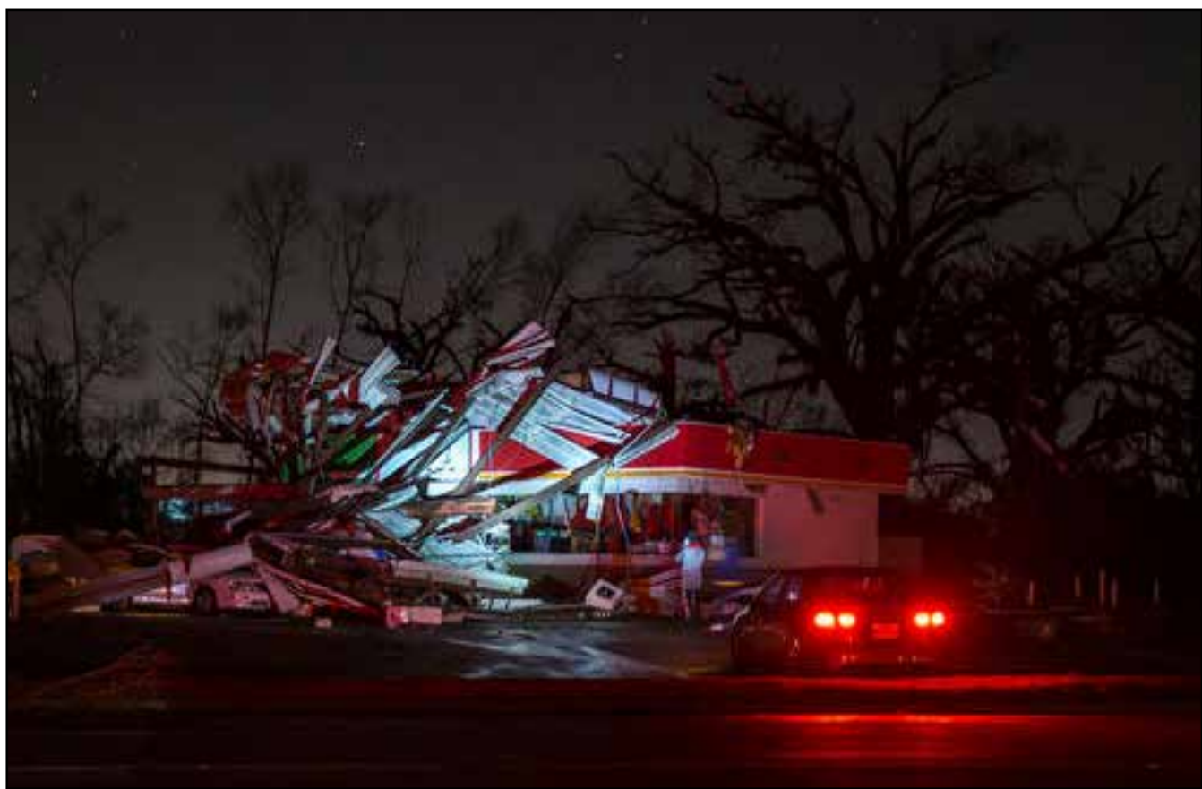
AP photo People stop to take a photo of a gas station damaged by an apparent tornado, Sunday, Jan. 22, 2017, in Albany, Ga. Nathan Deal declared a state of emergency in several counties, including Cook, that have suffered deaths, injuries and severe damage from weekend storms.
