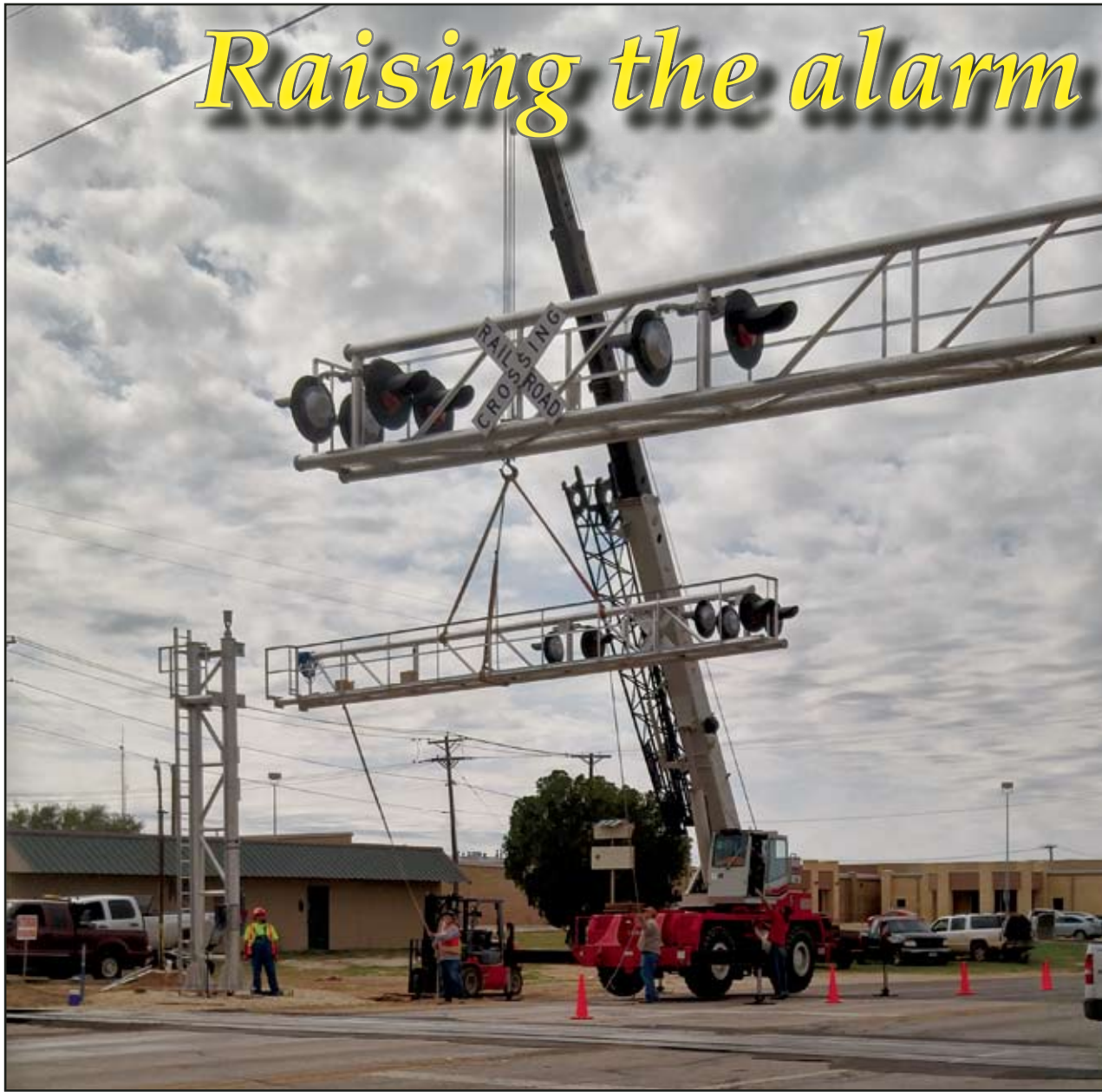
Crews were busy Friday afternoon installing a railroad crossing warning system where the rail spur crosses West Business 20 in Big Spring.
