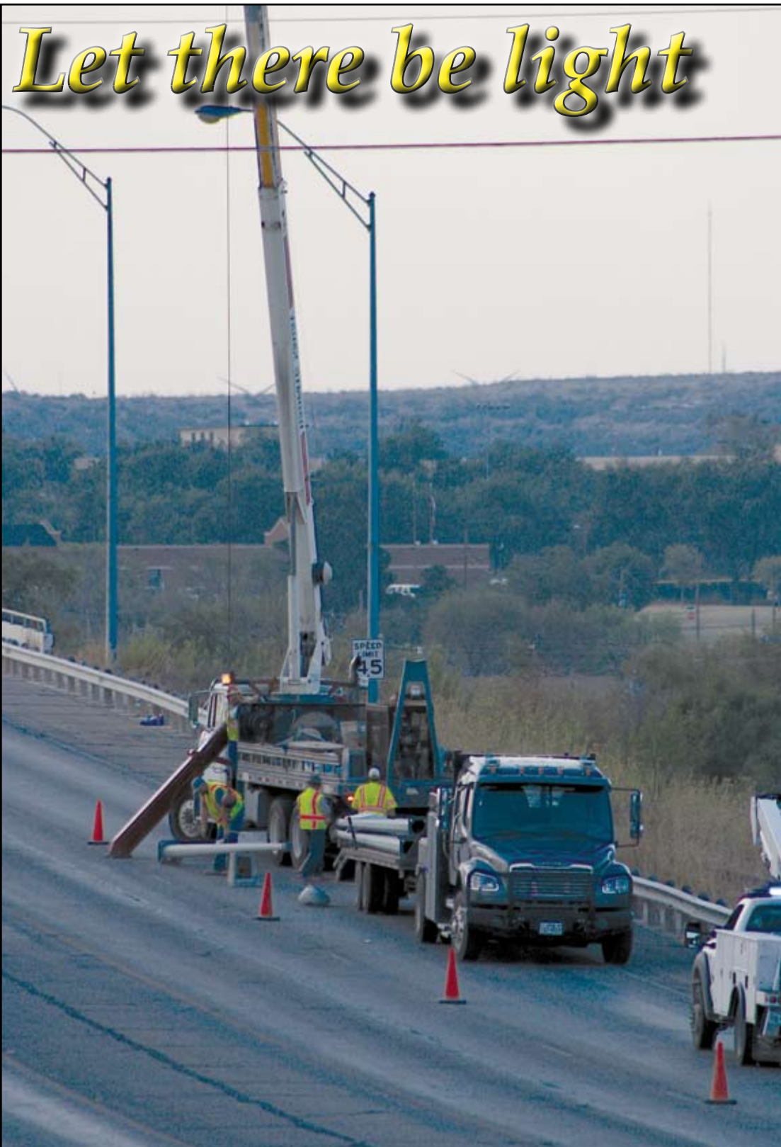
Texas Department of Transportation crews were busy replacing light poles along the Owens Street overpass Thursday morning.
