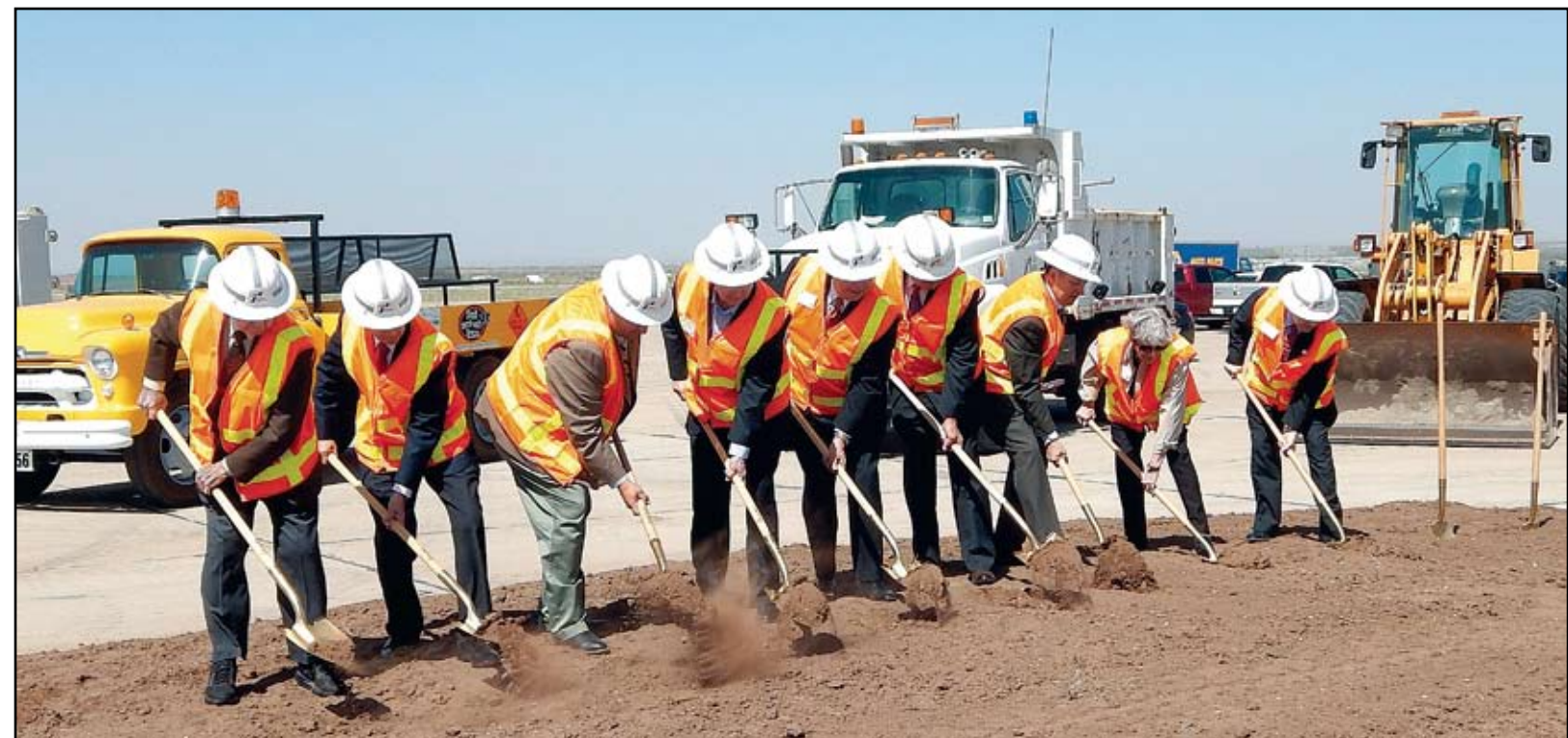
Dignitaries participate in groundbreaking ceremonies at McMahon-Wrinkle Airpark in April for the Highway 87 reliever route.
