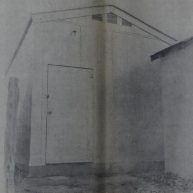
SHOWN in picture above is the outside of the new building which houses the equipment at the Nazareth exchange. West Texas Telephone Co. is having their open house December 3 and 4 so the public can view the new equipment now in use. —Staff Photo
