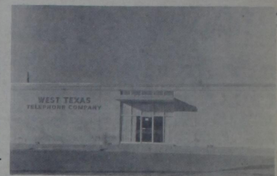
WEST TEXAS TELEPHONE CO. is celebrating their open house Friday and Saturday. The new central office is located at 113 N.E. 2nd. See story for details. —Staff Photo
