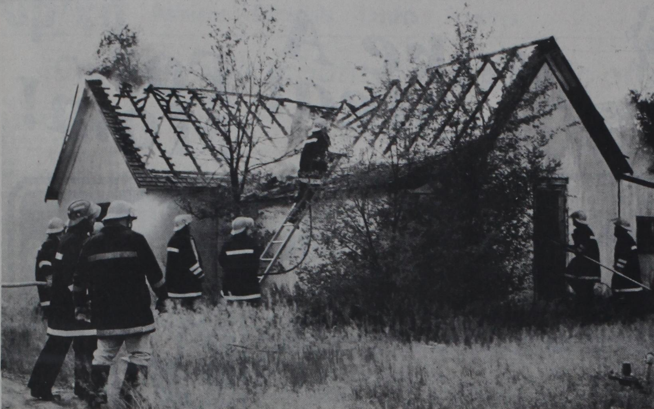
FIRE DESTROYED a vacant house at 107 NW Sixth in Dimmitt Tuesday afternoon. Two units from the Dimmitt Volunteer Fire Dept. responded to the alarm at about 5:15 p.m., but the entire house was aflame before firemen were able to arrive. Fire Mar-
