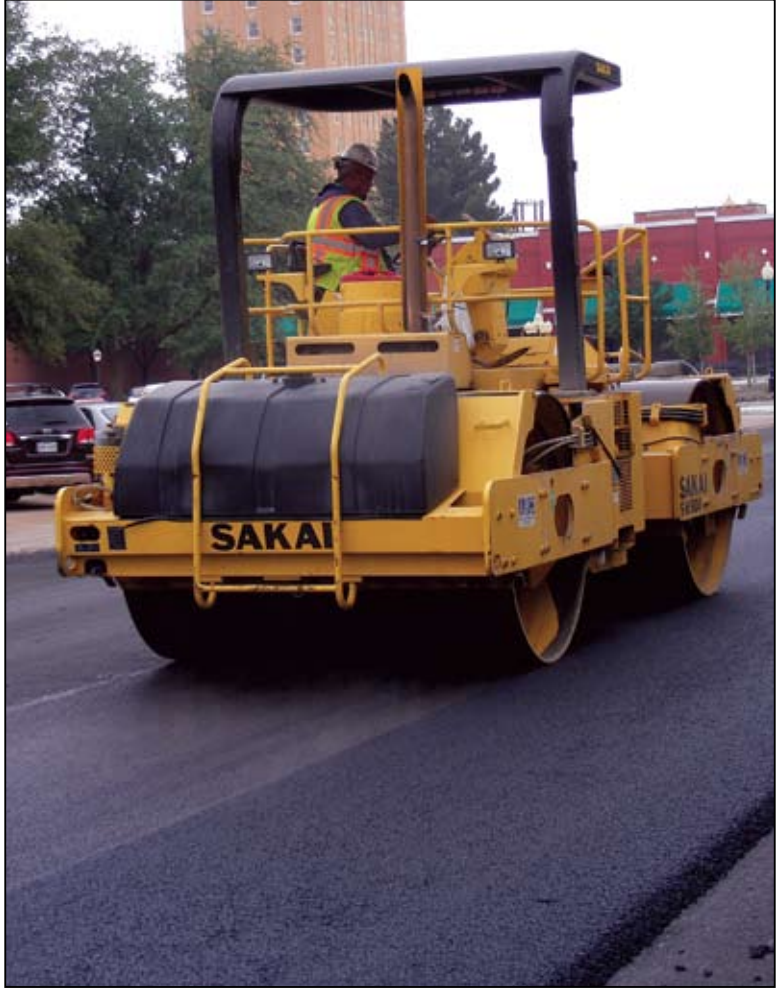
Clockwise, from top left: A "coal cow" machine collects asphalt mix used to pave the street; the machine operator gets a faceful of smoke; the "steel wheel" compresses the paving material to its desired thickness.
