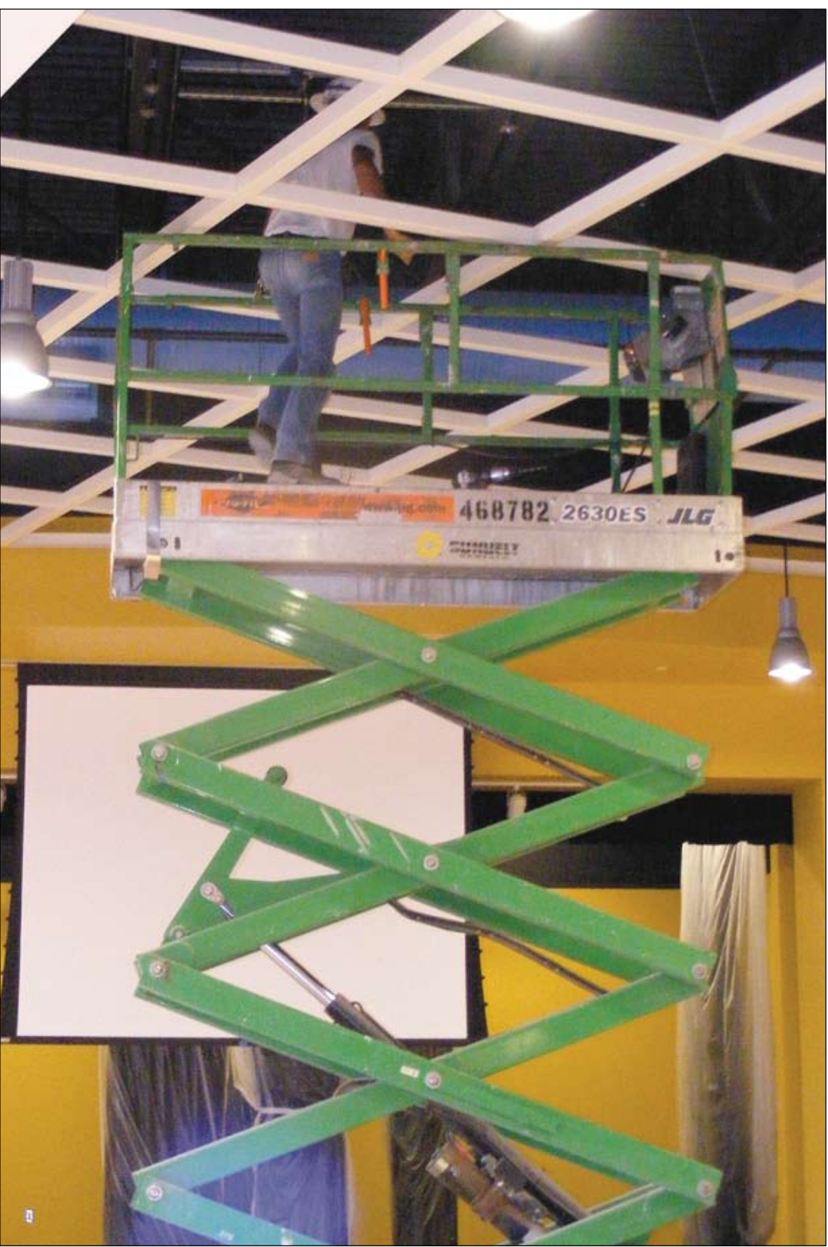
HERALD photo/Steve Reagan A worker uses a scissor lift to inspect the cafeteria ceiling area at the new Goliad Elementary on Wednesday afternoon. Four new elementary campuses will open to Big Spring students when the school year begins Aug. 27.
