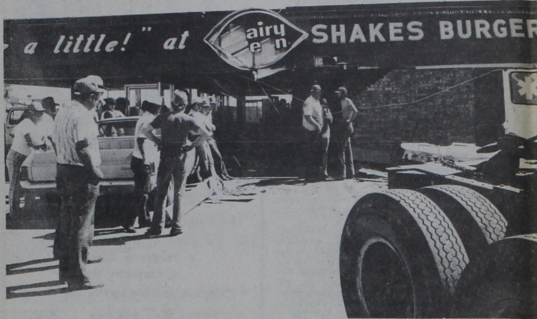
DAIRY QUEEN DEMOLISHED BY RUNAWAY TRUCK ... Freak accident left one seriously injured
