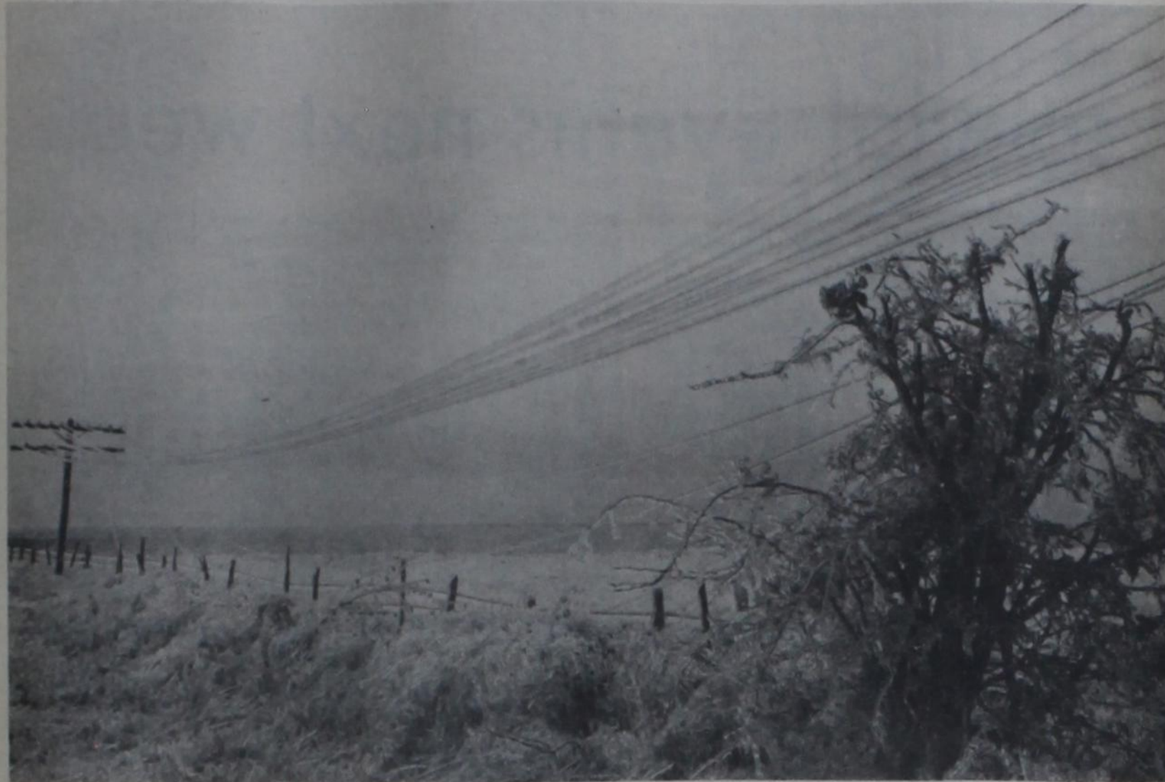
DOWNED UTILITY WIRES ALONG STATE 86 EAST OF DIMMITT ... Many poles also snapped, keeping repair crews busy
