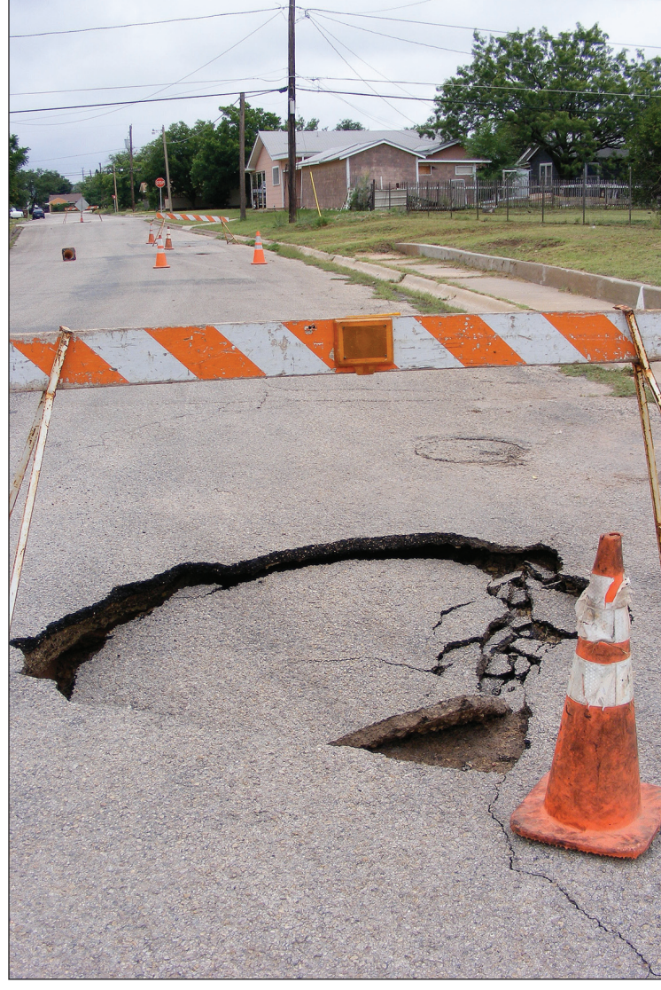
HERALD photo/Steve Reagan Subsurface moisture is considered the likely cause of a small sinkhole that appeared at the intersection of Bluebonnet and Rosemont streets this past weekend.
