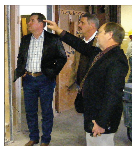
Howard College Executive Vice President Terry Hansen, right, discusses the renovation of the college's administration building with trustees Maxwell Barr, left, and Murray Murphy Thursday afternoon.
