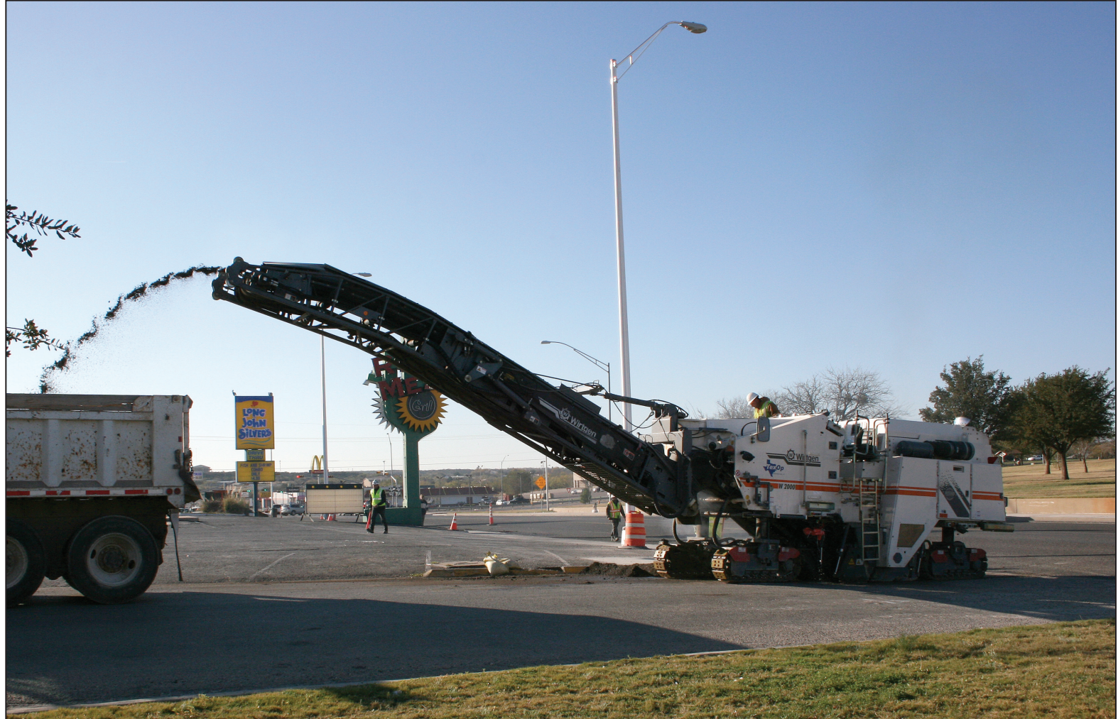
Construction crews mill a portion of the roadway on 24th Street between Gregg and Scurry early Monday morning, part of the Highway 87 street reconstruction project that has been ongoing for the past several months. Several roadways and intersections have been closed due to the reconstruction, causing numerous delays in traffic since the project began.
