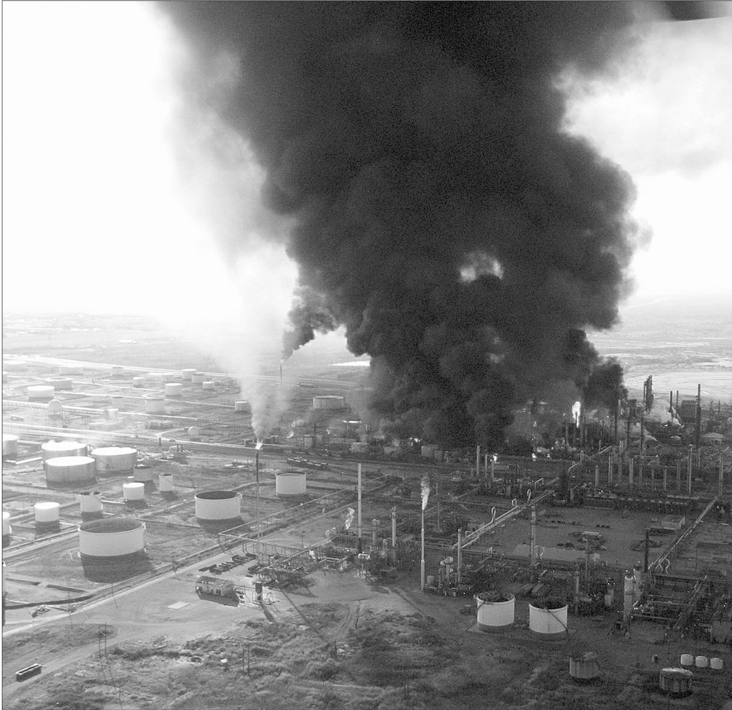
Smoke billows from fires that erupted at the Alon USA Big Spring Refinery Feb. 18. Despite extensive damage to the facility, no serious injuries were reported.
