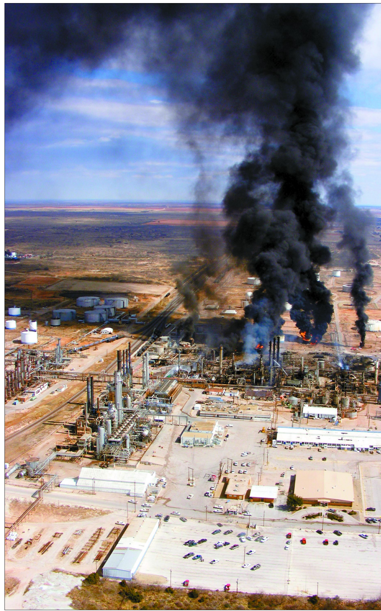
Smoke and flames roll out of the Alon USA Big Spring Refinery Monday morning following an explosion that rocked the facility. According to reports, the fire was caused by a leak in the refinery's propylene system. Fires were extinguished by late in the afternoon.
