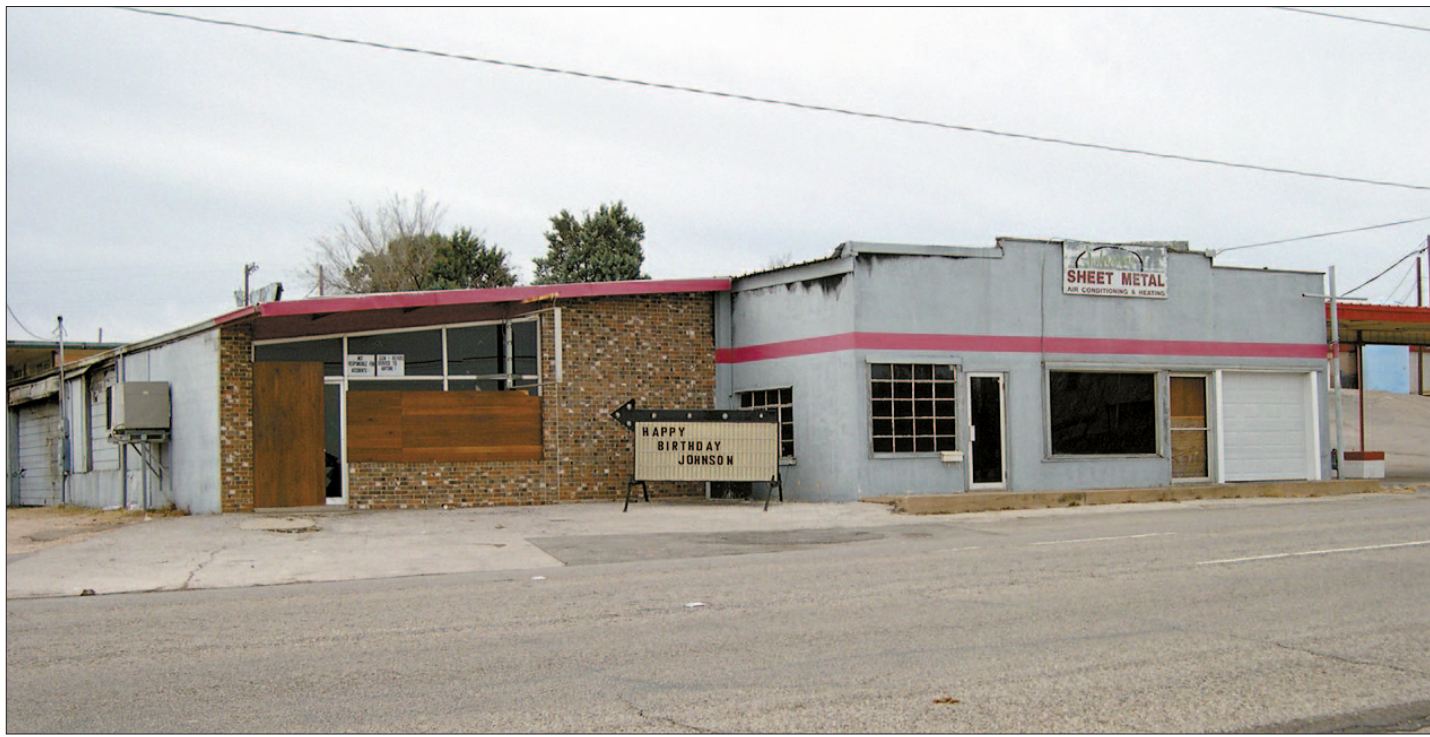
HERALD photo/Thomas Jenkins This structure in the 1300 block of Third Street was the scene of an attack by vandals early Monday morning, causing between $8,000 and $10,000 in damage when a vehicle being stored in the building was set afire. The incident is being investigated by the Big Spring Fire Marshal's office and the police department.
