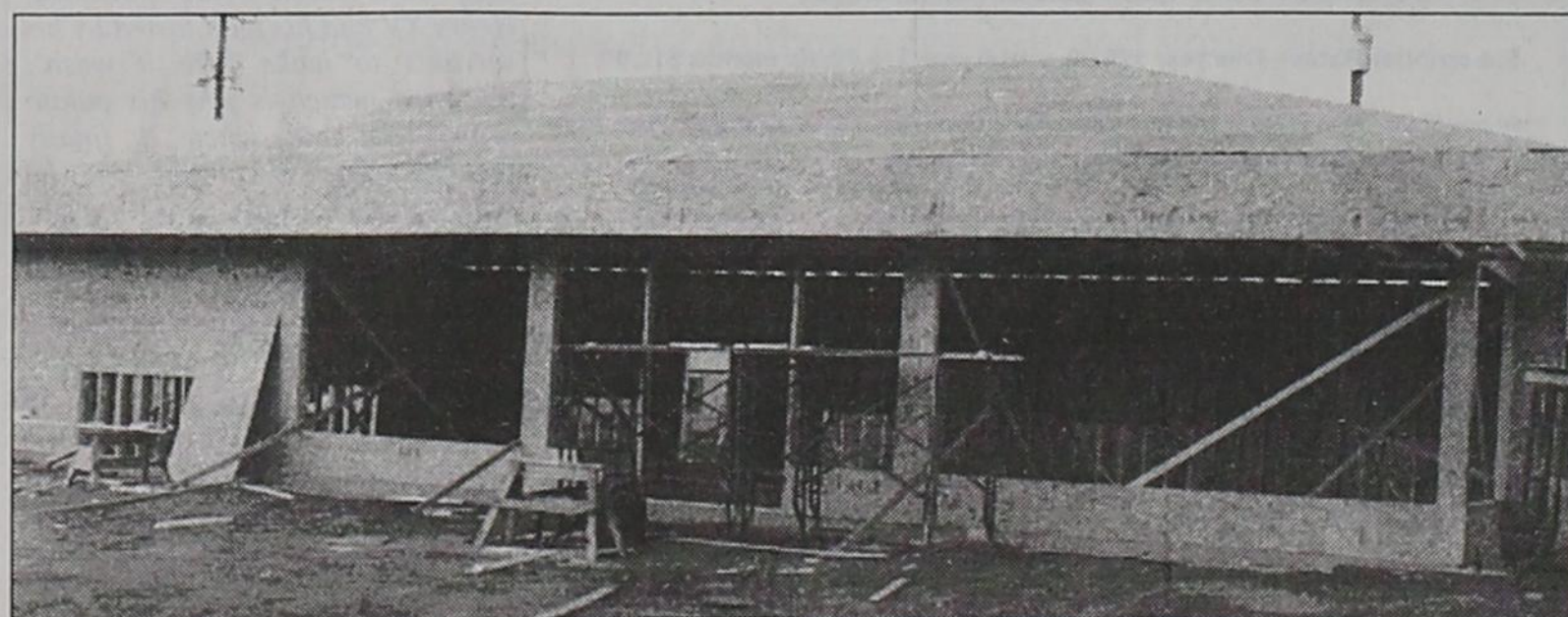
NEW CONSTRUCTION GOING UP
