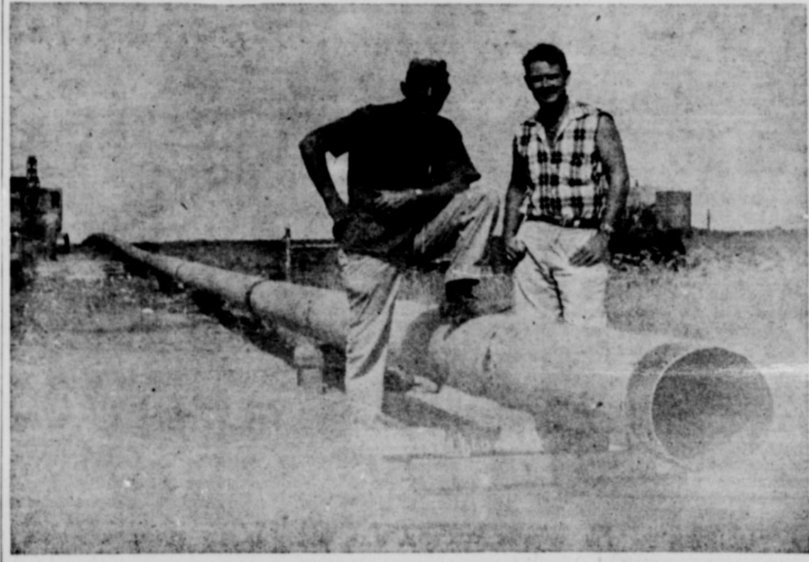
G. F. SMITH, left, superintendent with Vaughn & Taylor, Odessa, contracting firm in charge of laying the gas gathering system for the new absorption-type casinghead gasoline plant in northwest Yoakum County, is shown here with Jerry Taylor, inspector for the Honolulu Oil Company. The photo was taken out in the field and shows a portion of the 16-inch pipe ready to be laid. The plant, a multi-owned project, will be operated by the Honolulu Oil Company. —REVIEW Photo
