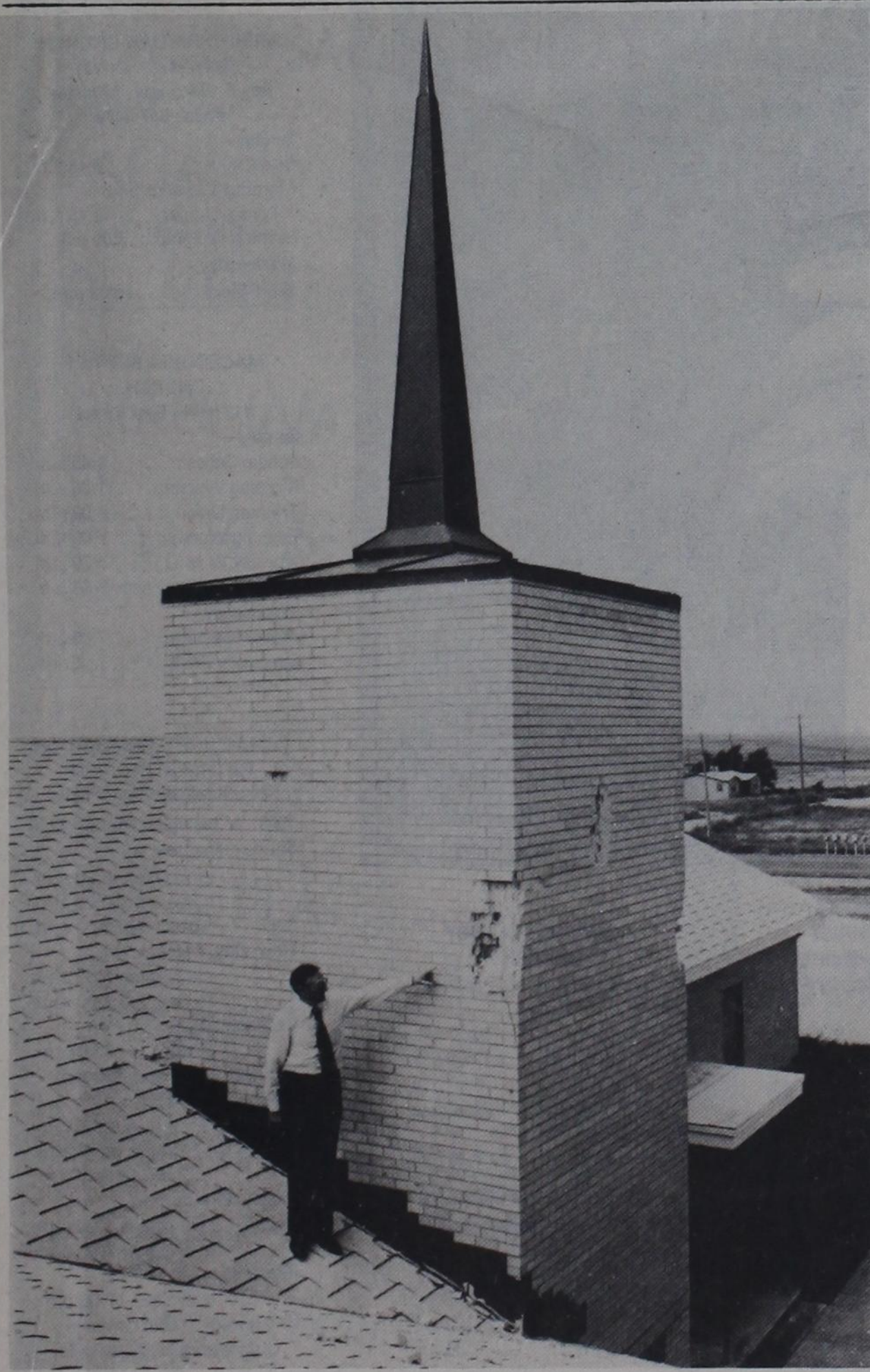
LIGHTNING STRIKES STEEPLE—Rev. Richard Clymer points to one of five places where a bolt of lightning exploded brick away from the steeple tower of the Sunnyside Baptist Church at 6:30 a.m. Tuesday. The lightning apparently struck the metal spire and cap first, then transmitted its energy to reinforcement
