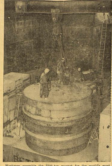
Workmen assemble the 2300-ton magnet for the world's most powerful cyclotron at Columbia University's new nuclear physics research center at Irvington, N. Y. The magnet, which contains more steel than a destroyer, will enable the cyclotron to smash even heavy atoms into 10 to 50 parts with new high energies of 400 million electron volts. The giant magnet is expected to start operating next summer.
