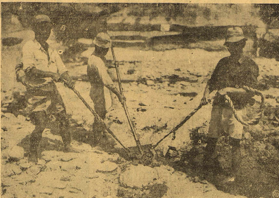
The camera of Richard C. Ferguson, NEA-Acme staff correspondent, caught about the last word in lazy labor near Seoul, Korea. Labor is so cheap and abundant that three persons often do a job that one could do alone. Typical is this shot of a ditch-digging trio. One merely holds and guides the long-handled shovel while his mates on either side use ropes to pull it along, then lift and dump it.
