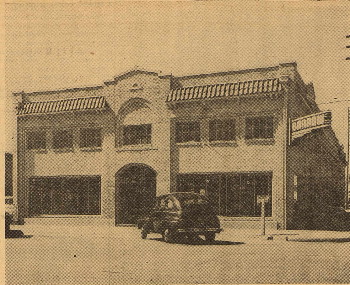
The Barrow Furniture Company, located at 123 North Loraine Street in Midland, is one of the finest and most completely stocked furniture stores in the Southwest. The business is housed in a spacious, modern and attractive building with large display windows and ample floor space. The firm, which caters to the every furniture need of citizens of Midland and the Permian Basin Area, has made every effort to maintain large and adequate stocks of quality merchandise for its many customers throughout this area. S. M. Vaughan is manager of the concern.
