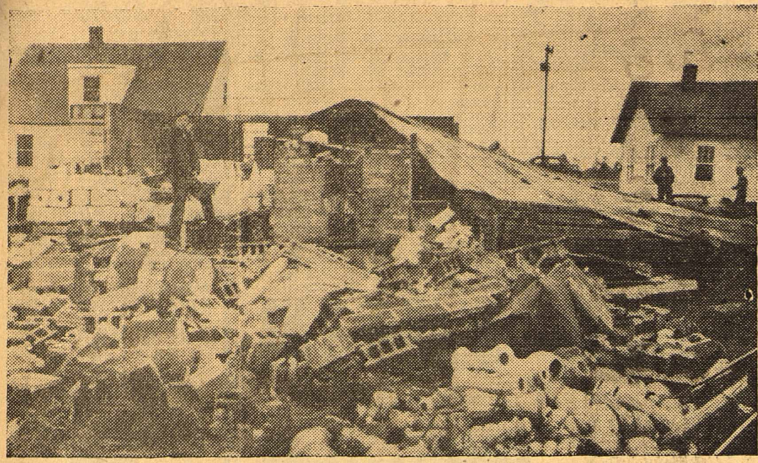
No "Bull in a China Shop," this, just a plain windstorm in Paris, Tenn., caused complete destruction.
