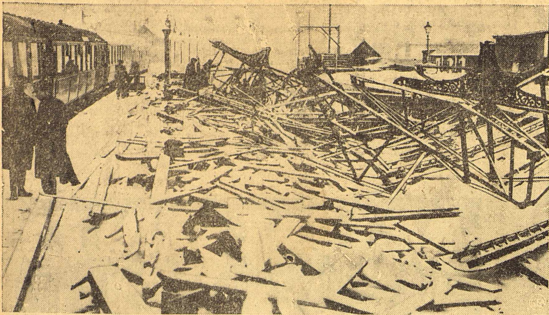
Victim of one of England's worst blizzards in 30 years is the railway station at Grantham, Lincolnshire. Just after express train thundered through, tremendous weight of snow caused station roof to collapse on tracks, as pictured above, blocking traffic for some time.
