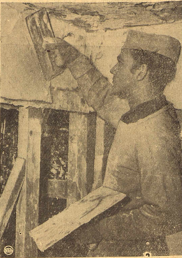
Navy veteran Norman C. Nusser, 22, a deft man with a hawk and trowel. Since graduation from pre-apprentice school last October, he has worked on four houses and two larger buildings.
