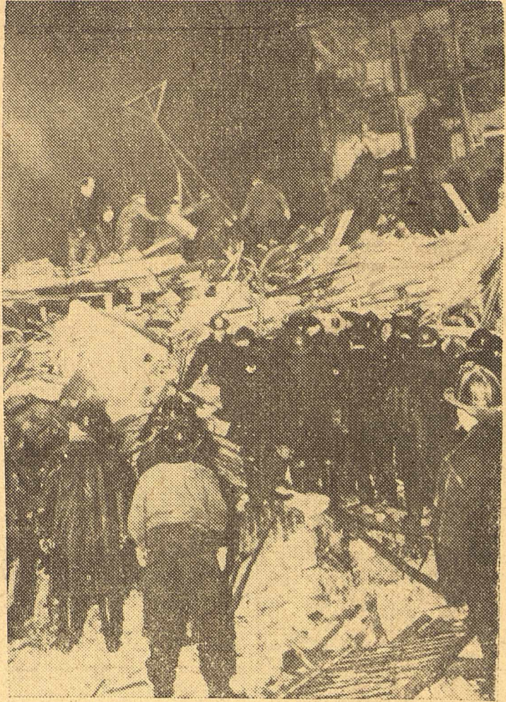
(NEA Telephoto) Firemen dig into the wreckage for victims of an ice-house fire, which caused an entire rear wall to collapse on a 27-family tenement in New York City. Twenty-one are known dead and 15 are missing.
