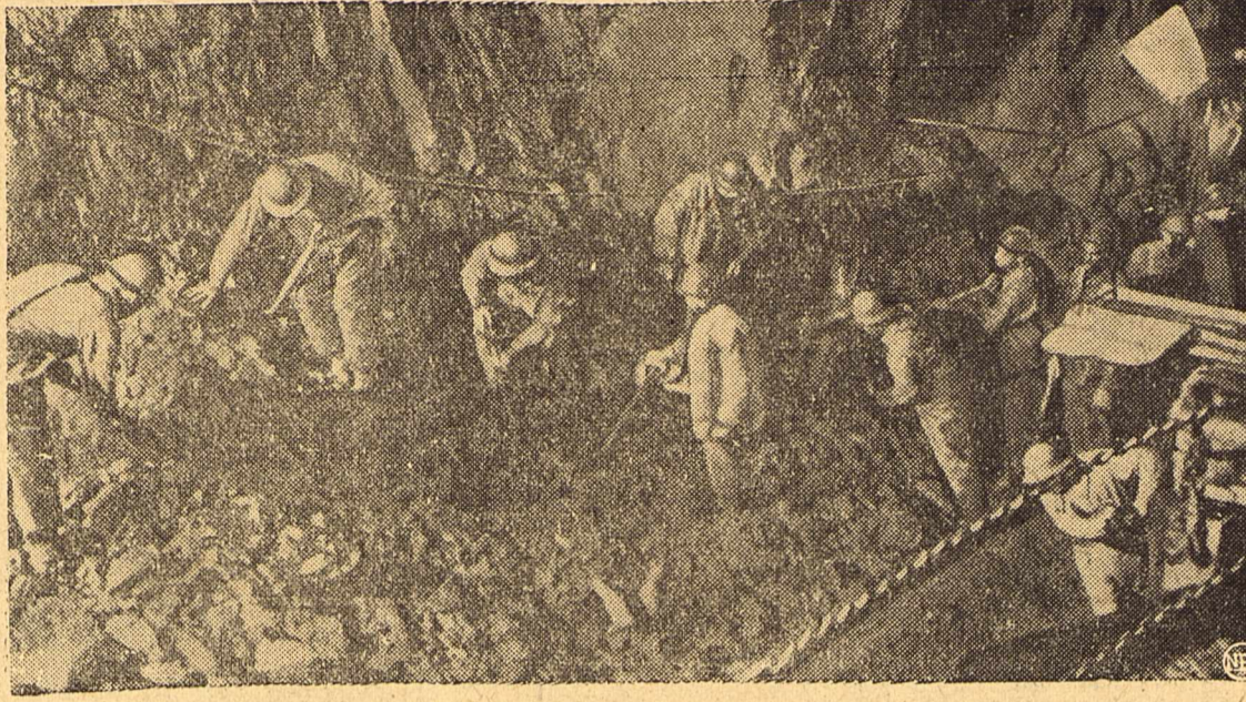
Human moles: Sandhogs at work make this eerie picture as they shovel rock and muck, which has been blasted from the face of the Brooklyn-Battery tunnel, into "mucking machine".
