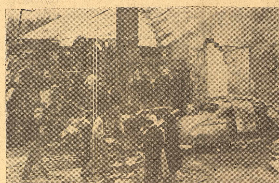
(NEA Telephoto) This is what is left of the Warrenton, Mo., bus station after a 1000-gallon tank of cooking gas exploded. Detonation was very violent, killing two persons and injuring five others. Windows were broken 100 yards away.
