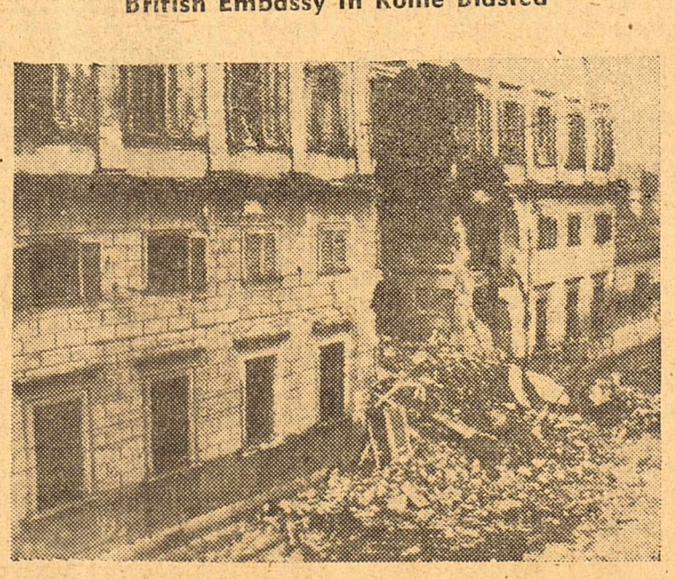
(NEA Telephoto) Damage to the main entrance hall of the East Wing of the British Embassy in Rome is shown in this radiophoto. The blast, believed caused by explosives left on the steps of the embassy in two suits, occurred early Thursday.
