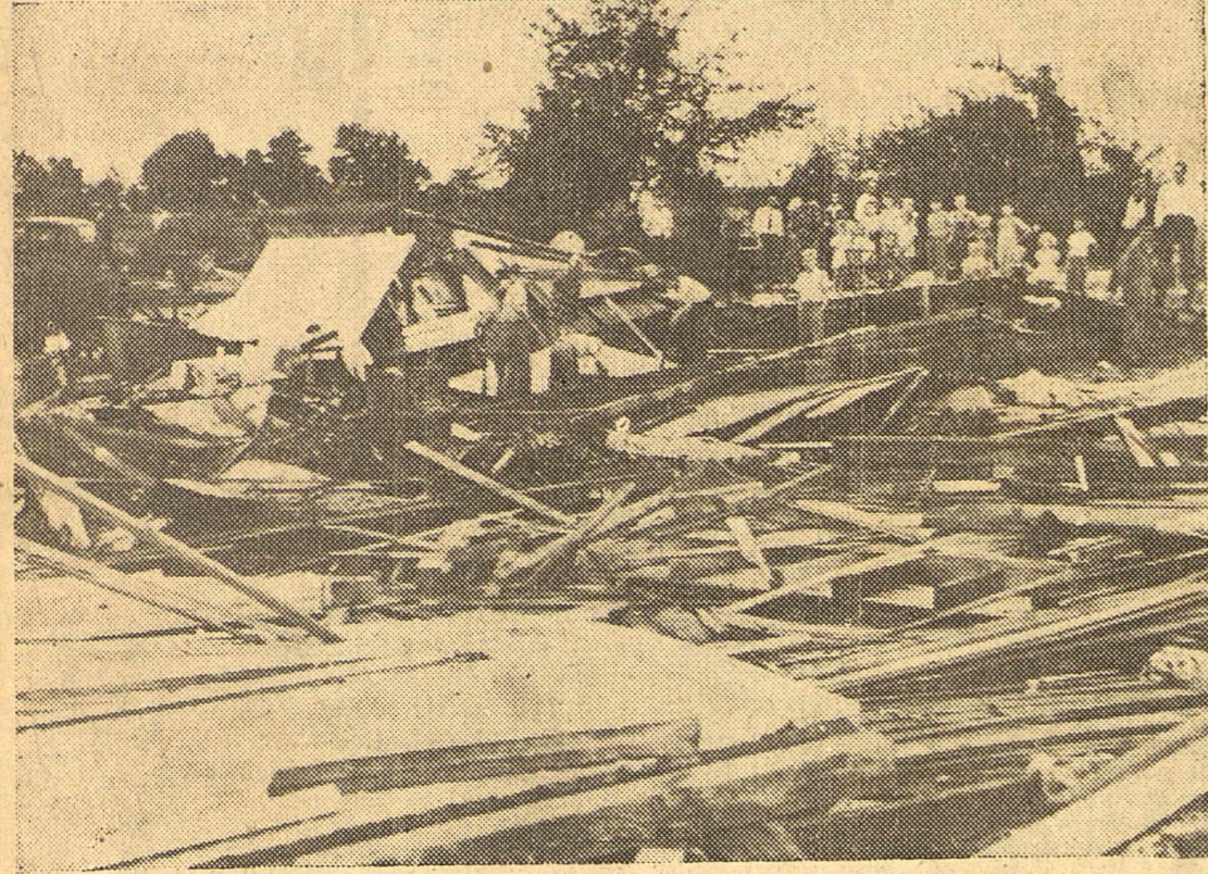
Curious residents of Austell, Ga., look at the wreckage of one of the homes destroyed by a freak tornado which injured four persons as high winds blew down several buildings. (NEA Telephoto)
