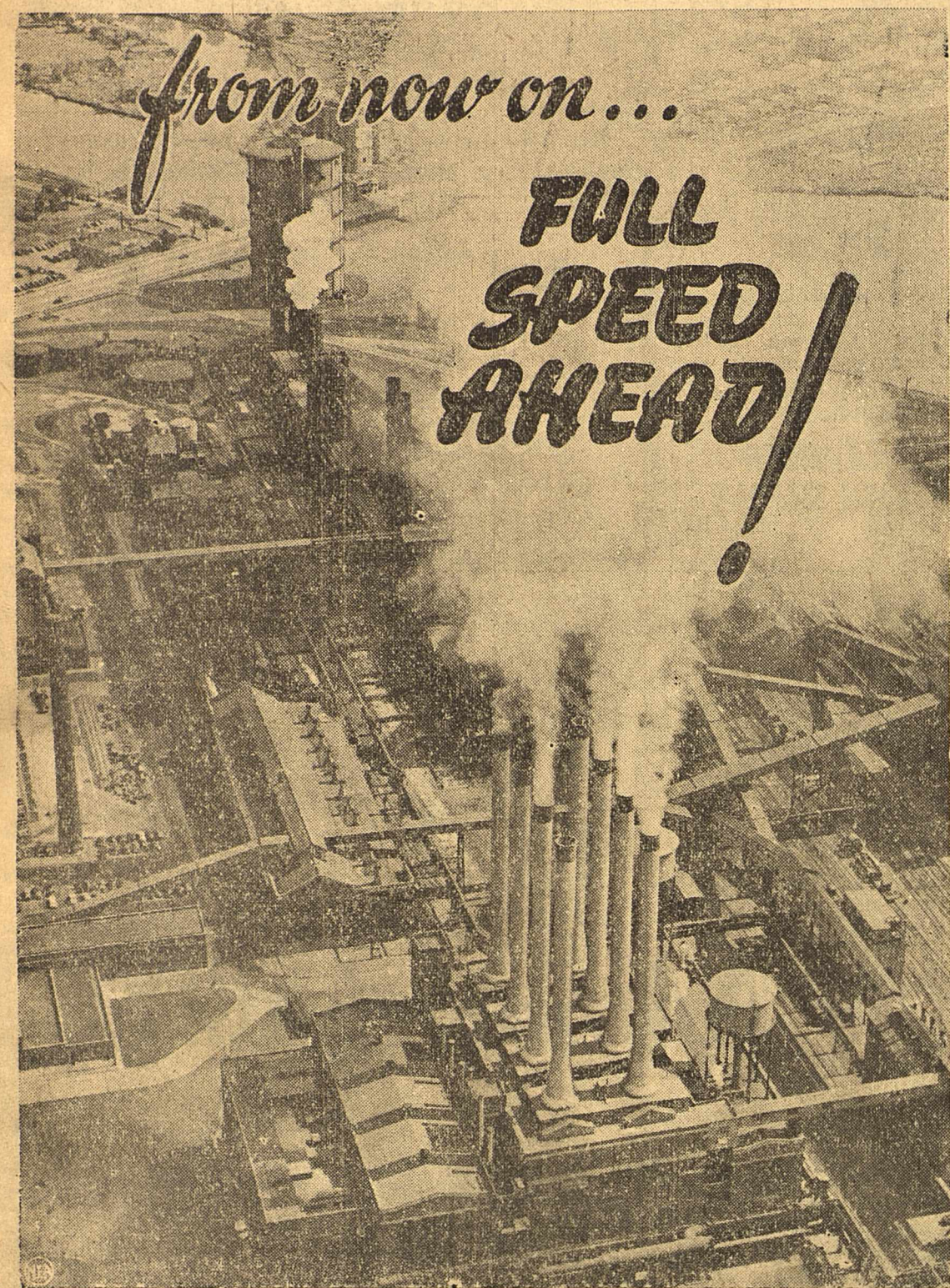
Let America's myriad industrial chimneys send up billowing smoke signals that bespeak all-out peacetime production, symbolized by the dramatic airview, above the great Ford plant at River Rouge, Mich.
