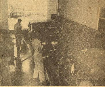
Wash and steam cleaning room, 2-car capacity. High prsesure washer, soft water for rinsing. Latest type steam cleaner
