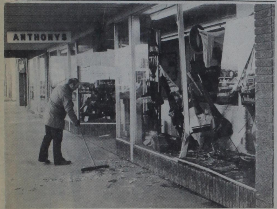
SWEEPING UP is C. R. Anthony's manager Leroy Maxwell after an unidentified driver ran into the store's front last Thursday around 6 a.m., breaking two large sections of the
