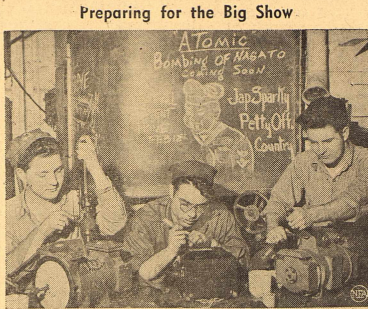
With artistic attempts by fellow crewmen as a background, Electrician's Mates 3/c John D. North of Detroit, Mich.; Charles L. McCreery of Onaway, Mich., and Thomas Callahan of Mechanicsville, N. Y., repair motor parts aboard the Jap battleship Nagato. The ship will be a target in atomic bomb tests in the Marshall Islands area of the South Pacific in May. Photo by Tom Shafer, NEA-Acme correspondent.
