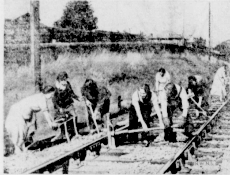
Road gangs made up of men have a tough job ahead. It was difficult some time ago to imagine women doing this rough work on the railroads, but that's what they are doing now in Great Britain. Women surfacemen are jacking up and packing the railway lines, using muscle and technique in the same fashion as the men.
