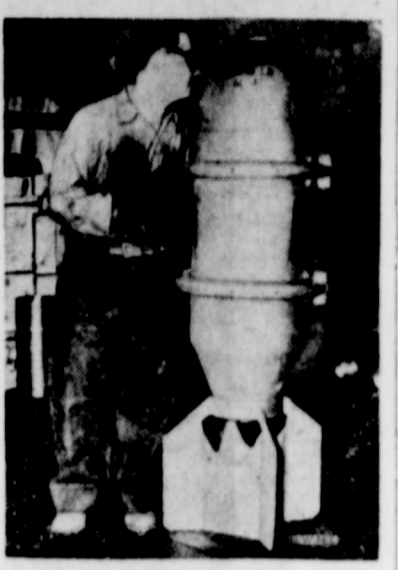
Ready for shipment to an ordnance department loading plant to be filled with explosive, this 500-pound demolition bomb is getting a final examination in a bomb manufacturing plant at Philadelphia. Pins were attached for photographic purposes. Ordinarily bomb pins are attached at air fields.
