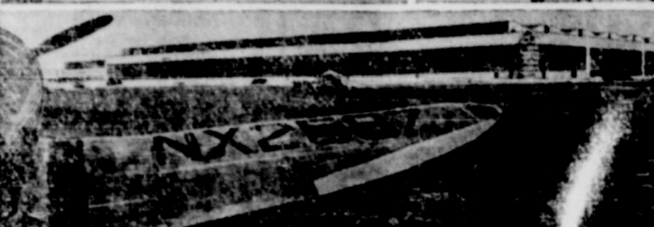
Assembly building for Republic Aviation Corporation, Farmingdale, N. Y. Steel was erected in two months and two days.
