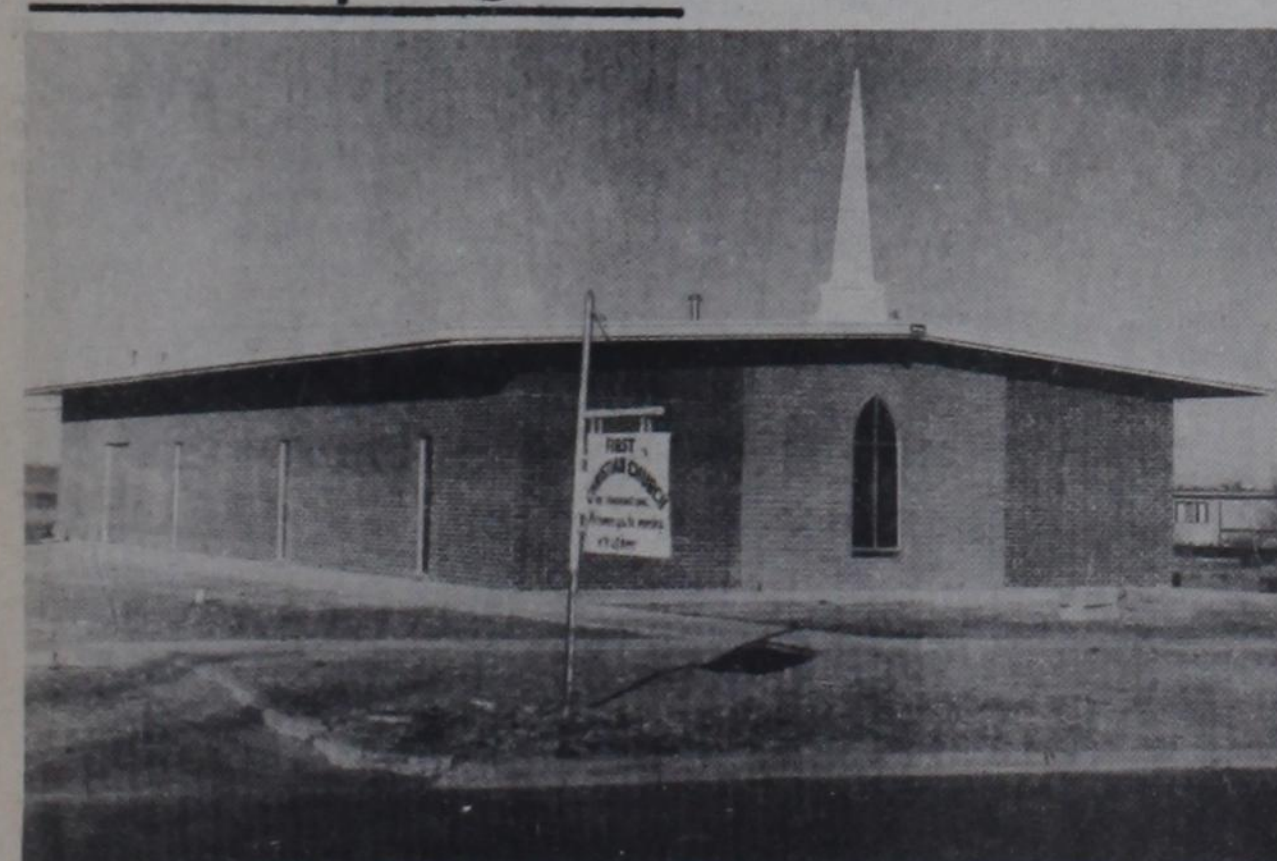
FIRST CHRISTIAN—Members of the First Christian Church of Dimmitt held their first worship service in their new building on Western Circle Drive Sunday morning. Although it's a steel building, the only steel visible is in its roof. Inside, the new building
